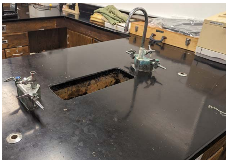
1966 High School science labs equipment and furnishings are worn and need replacement.
